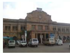
Nagpur Railway Station
